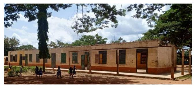
This project is meant to re-roof the 4-unit classroom block, strengthen the columns, repair the floors of the classrooms and veranda, fix the damage windows and doors, provide ceiling to the classrooms, electrical installation, supply textbooks and provide teacher fresher training to the teachers to enhance teaching and learning and improve upon learning outcomes. The total cost of the project is estimated at **USD30,300. Minimum for global grant.**
